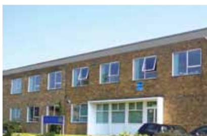
UK Headquarters in Harlow, United Kingdom. Harlow is home to administration, test facilities and laboratories.
