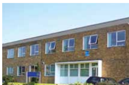
UK Headquarters in Harlow, United Kingdom. Harlow is home to administration, test facilities and laboratories.
